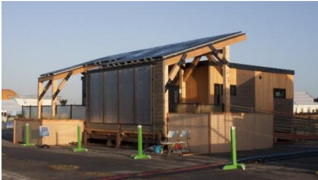
The ECHO exostructure as seen from the southwest
