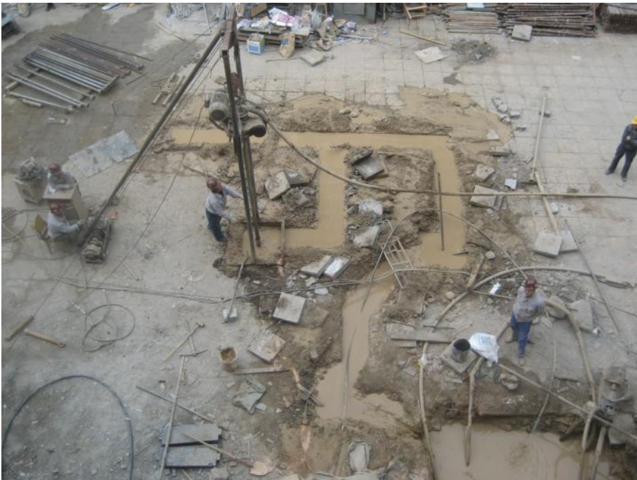
Drilling boreholes for CABR's new near NZEB
